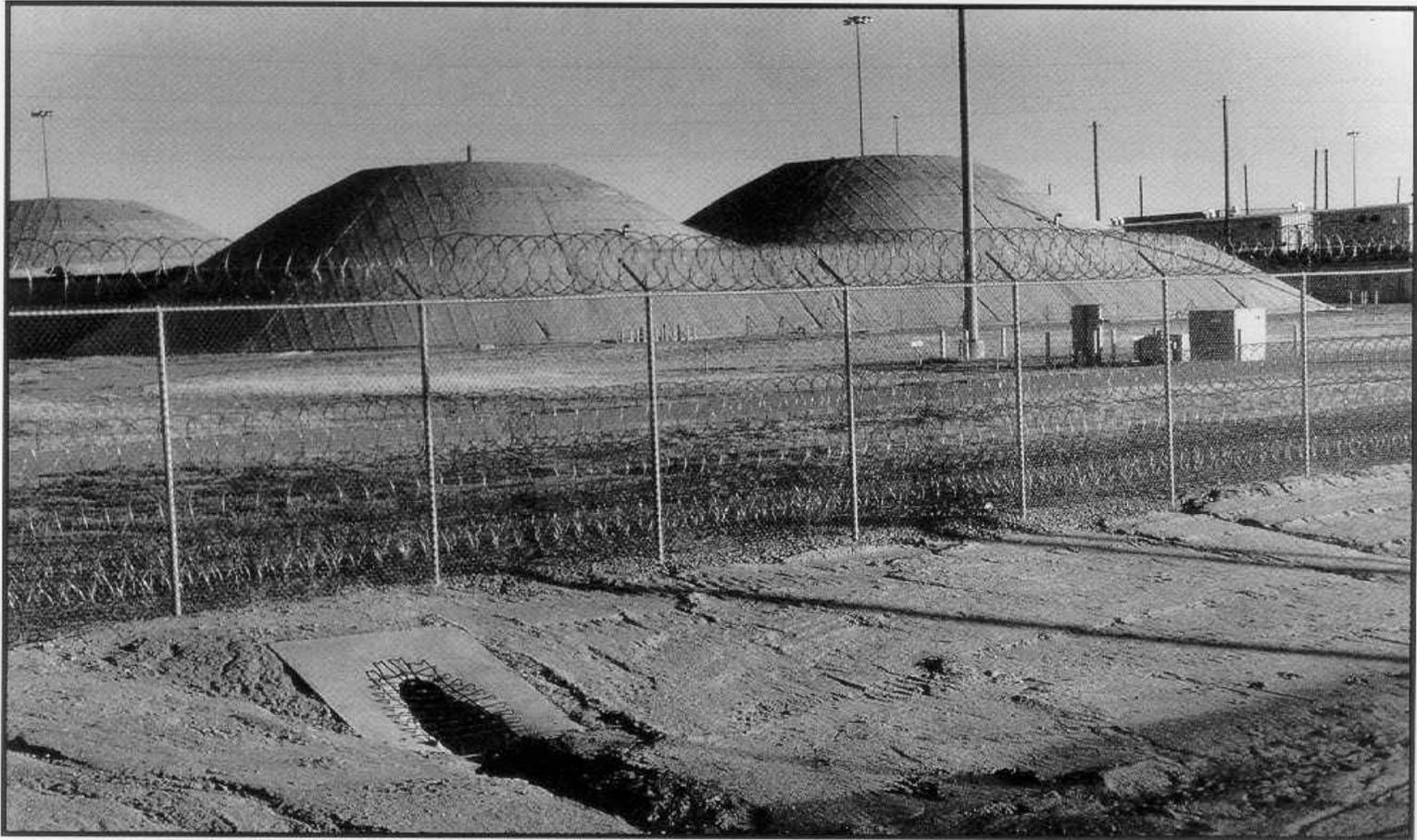
**“Gravel gerties”** are concrete structures whose roofs consist of cable mesh supporting large amounts of gravel. Beneath them are bays, where workers assemble and disassemble nuclear warheads. Should a warhead’s conventional explosives accidentally detonate, the roofs of these structures are engineered to give way, releasing the gravel and trapping the plutonium particles. Up to 2,000 warheads per year are now being dismantled at this site. *Pantex Plant, Amarillo, Texas. November 18, 1993.*
