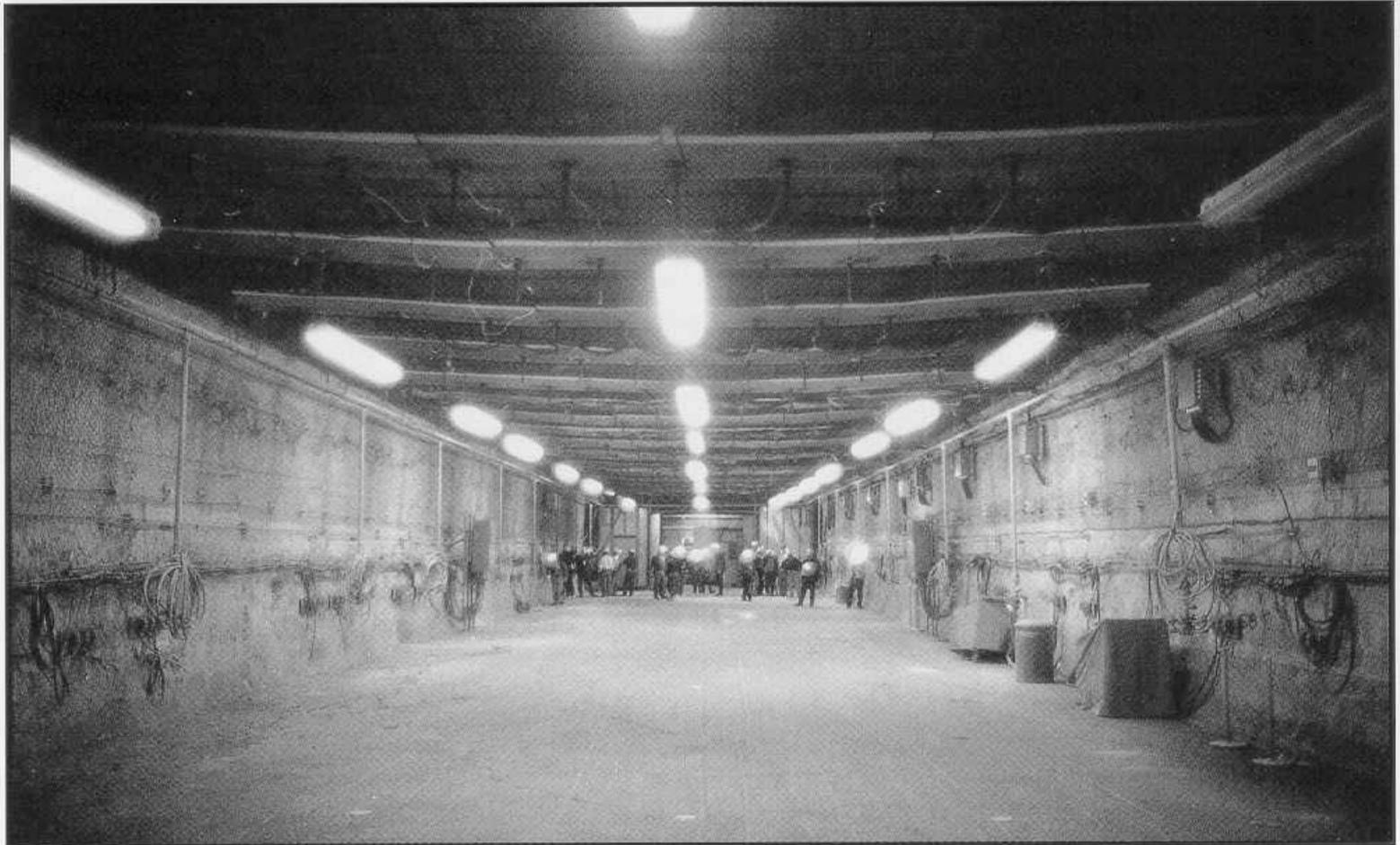
**This underground waste-disposal room**, excavated in 1986, was the first of 56 chambers to be excavated at the WIPP. It is 300 feet long, 33 feet wide, and 13 feet tall and could hold six thousand 55-gallon drums of transuranic waste. It lies 2,150 feet below the surface of the earth. *Room 1 of Panel 1, Waste Isolation Pilot Plant, near Carlsbad, New Mexico. February 25, 1994.*
