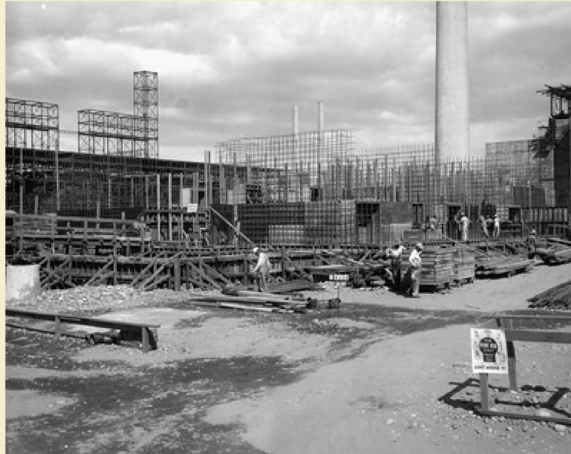
Hanford Site Construction
