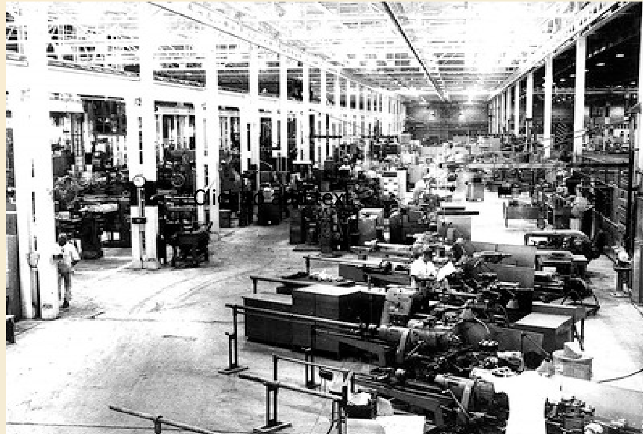
Oak Ridge Gaseous Diffusion Plant – Machine Shop
